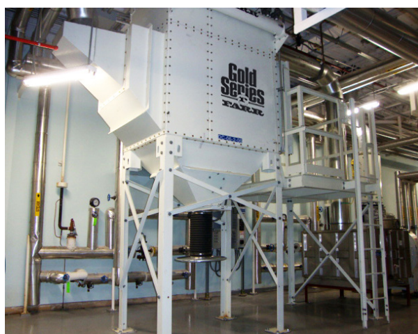
Example of an installation of a typical dust extraction/ collection system
