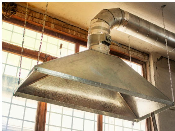
Hoods over work area captures dust and fumes .
