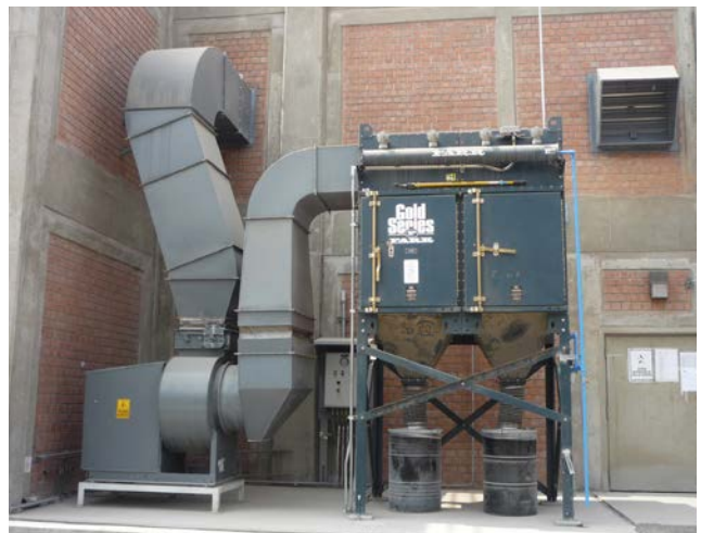
A 16-cartridge dust collector pressurizes and ventilates a compressor room in a power generation plant. Wall louvers allow for air exchange and are calibrated to maintain a specific pressure inside the facility.
