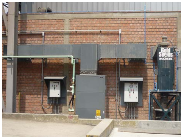
A small cartridge collector is used to pressurize an electrical room. Located in a warm climate, the room has its own backpack-type A/C unit for cooling, and the dust collector is sized for 10 percent of the capacity of this unit.
