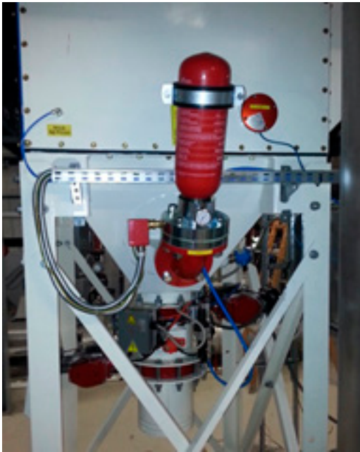
Figure 6 - A collector protected by suppression
