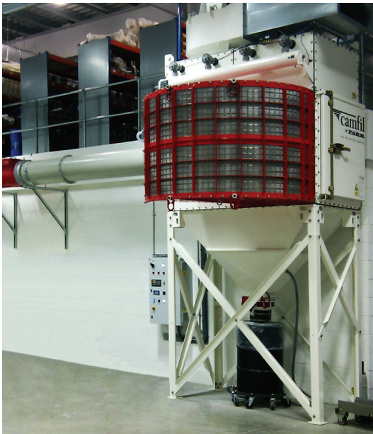
Figure 4 - A dust collector with flame quench
