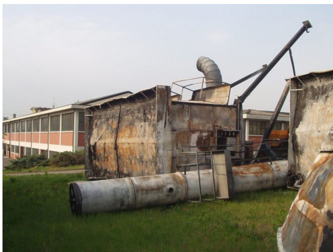
Figure 1 - Dust collectors after a catastrophic explosion
