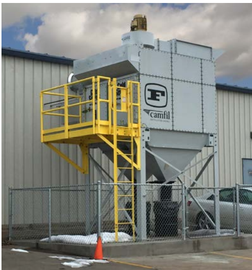
A Farr Gold Series® 20-cartridge collector captures fumes from three automated flat laser cutting machines.
