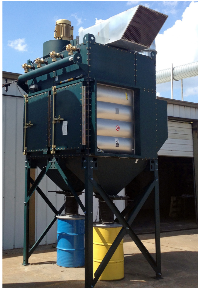
Dust collector used on a spray and fuse application incorporates an explosion vent and isolation valve due to the combustible material in the spray process.
