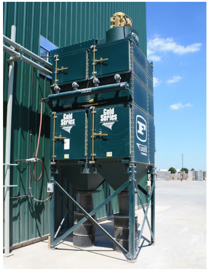
Dust collector designed for silica dust capture to meet OSHA's stringent new silica rule.
