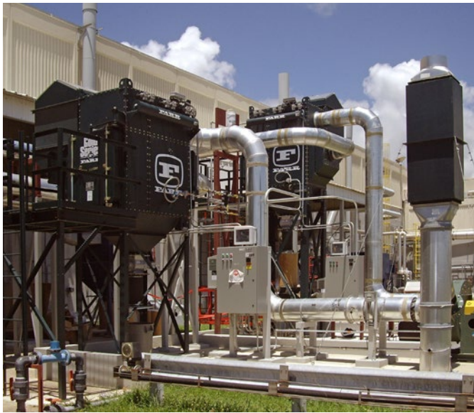
Pharmaceutical processing facilities like this one are among those most likely to be impacted by Standard 199.
