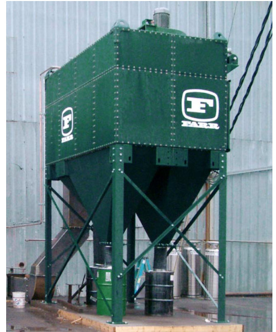
Farr Gold Series® GS24 installed at Chatham Steel on a plasma cutting table application.
